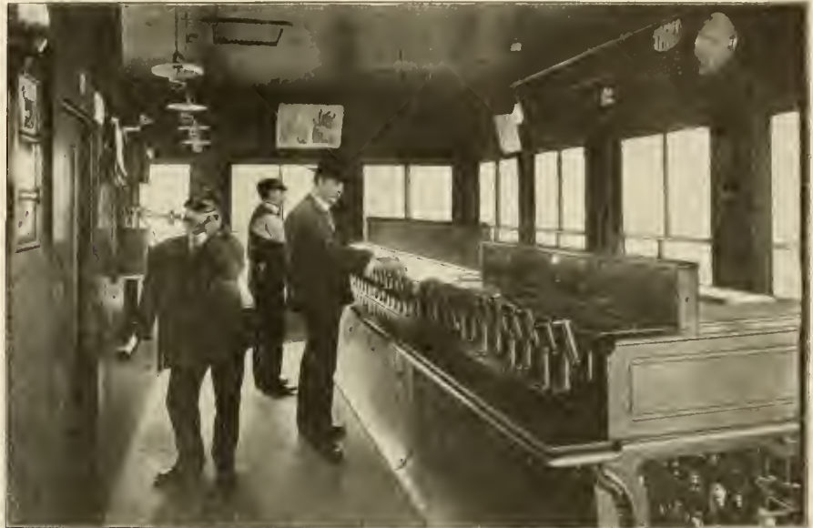
INTERIOR OF SIGNAL TOWER AT OAKLAND, CAL., SOUTHERN PACIFIC.
